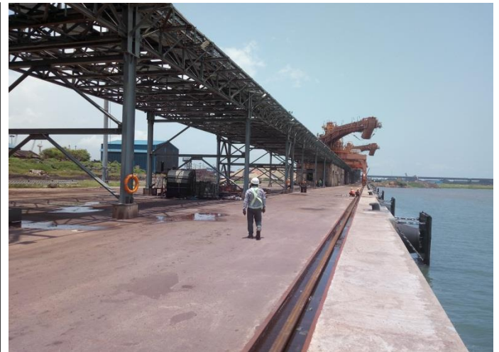
CONVEYORS & SHIPLoadERS (7000 TPH EACH FOR 180,000 DWT SHIP) UNDER INSTALLATION ON THE BERTH. BERTH CONSTRUCTED ON SHORE BEFORE COMPLETION OF FRONT DREDGING, WHICH IS IN PROGRESS
