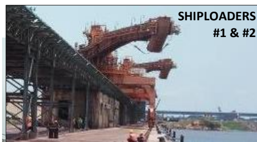
CONVEYORS & SHIPLoadERS (7000 TPH EACH FOR 180,000 DWT SHIP) UNDER INSTALLATION ON THE BERTH. BERTH CONSTRUCTED ON SHORE BEFORE COMPLETION OF FRONT DREDGING, WHICH IS IN PROGRESS
