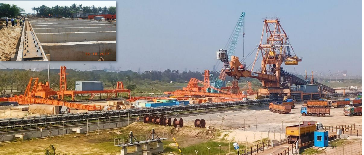
STACKER-RECLAIMER (4000/7000 TPH) FOR IRON ORE STOCKYARD UNDER ERECTION. STORAGE YARD UNDER CONSOLIDATION & CONSTRUCTION
