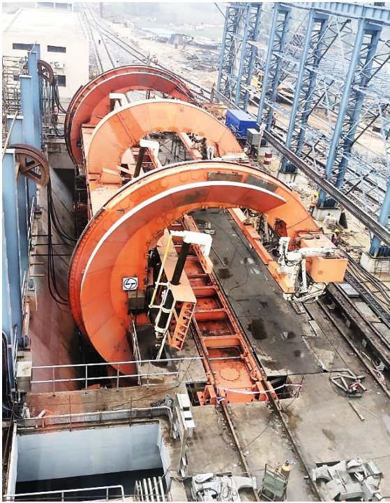
BOTH TANDEM AND SINGLE WAGON TIPPLER STATIONS UNDER ERECTION
