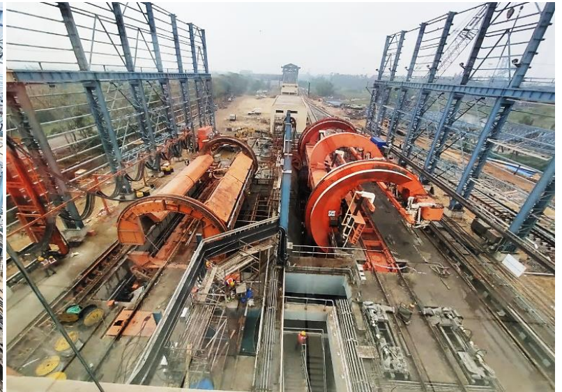
BOTH TANDEM AND SINGLE WAGON TIPPLER STATIONS UNDER ERECTION
